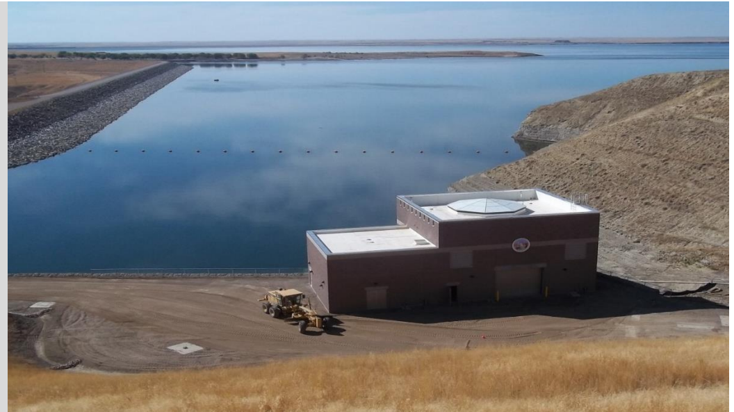
35 MGD Wet Well Pump Station Chester, MT
